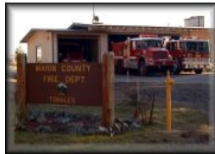
Tomales Fire Station
