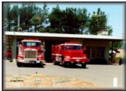
Hicks Fire Station
